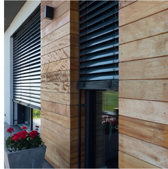
Facade blinds, view from the outside
